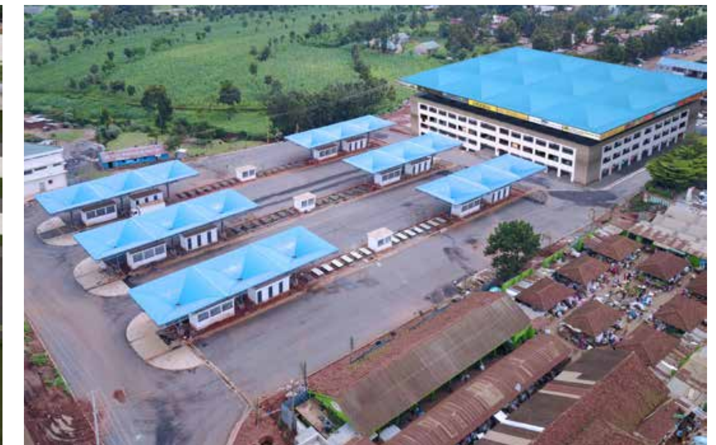
Aerial shot of actual site under construction
