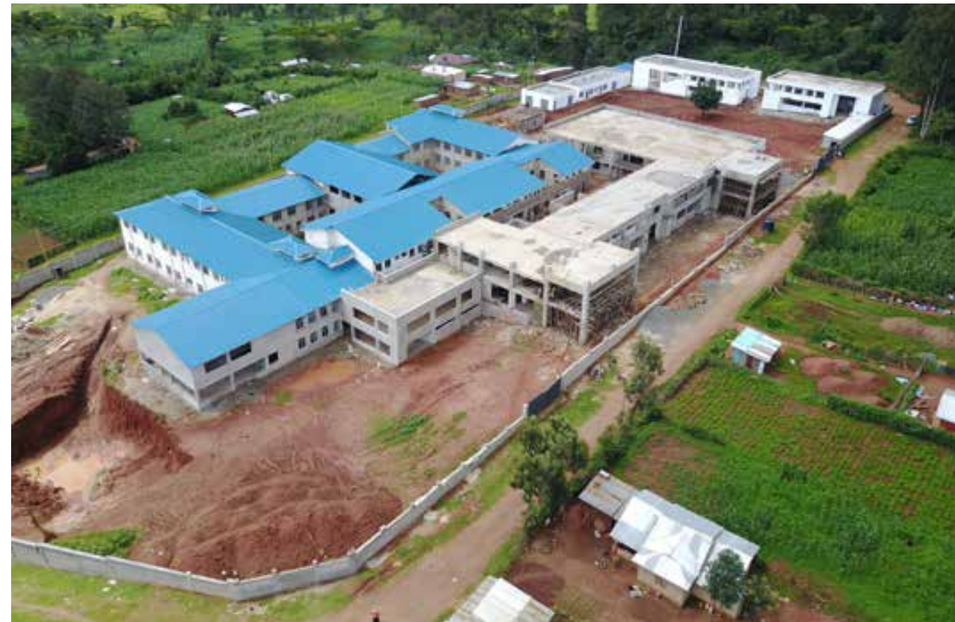
Aerial shot of actual site under construction
